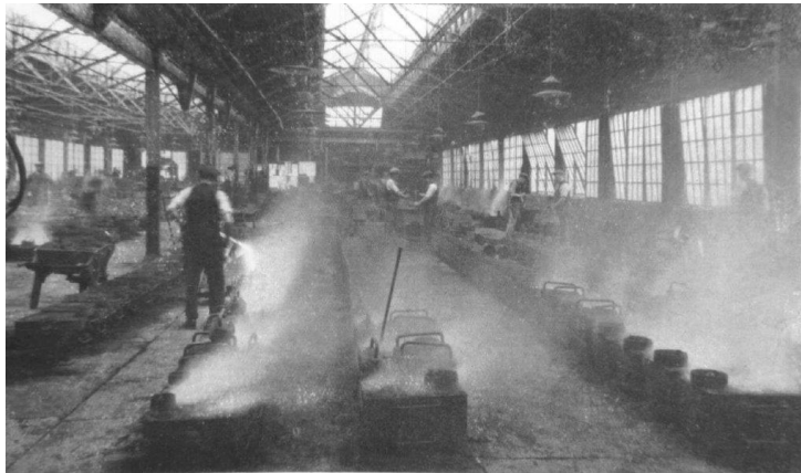
The Rail Chair Foundry, Swindon Railway Works. The foundry man is pouring molten iron into moulding boxes to cast rail chairs, these fixtures hold the railway line to the sleepers.
